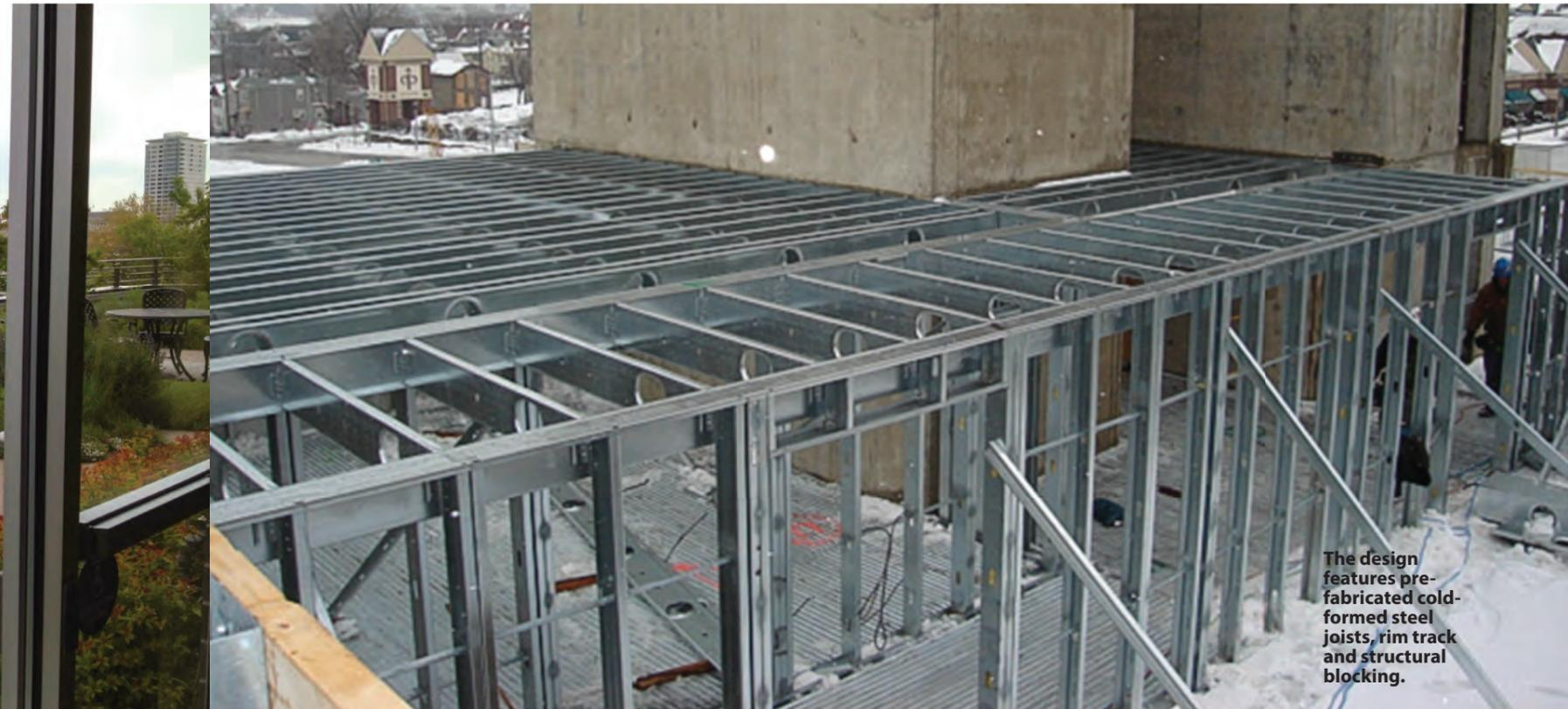
The design features pre-fabricated cold-formed steel joists, rim track and structural blocking.
